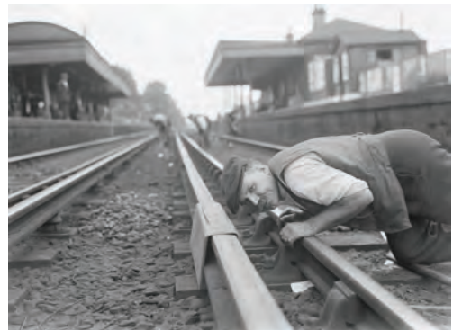
A railway worker gauging the lines in Sidcup, Kent. 1937
